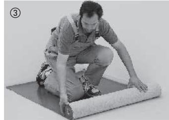
③ For sound insulation and to smooth out slight irregularities of the subfloor, unroll 2 mm thick luxury insulation layer. Our range of accessories also offers suitable insulation underlays. Asphalt-bitumen felt and carpeting is not suitable for sound insulation. **Parquet with integrated insulation layer is not suitable for glue-down installation.**
