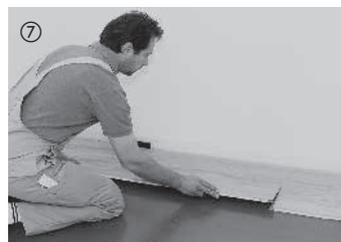
⑦ The next row is started with the leftover piece of the first row (short side offset of at least 50 cm). This considerably reduces waste. The rest of the installation is performed board-by-board. First, the boards are angled into the previous row along the long side by applying a small amount of force. Tap edge gently with tapping block, if necessary.
