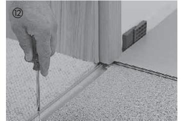
In doorways, mount a suitable moulding system to ensure the necessary expansion space. This also applies if the same floor is to be laid in the adjoining room. In this case, a transition moulding should be used for covering the required expansion gap. Leave an expansion space of approx. 5 mm between the board and the base of the moulding. As a rule, a fine saw must be used to cut a gap the thickness of a board in wooden door frames to allow the parquet to expand.
