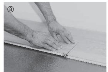
⑧ The board is then lowered in on the short side. Ensure here that the board is flush at the short side with the previously laid board. Pressure applied briefly to the side joint clicks in the board.
