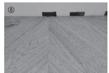
In the wall area, fit in cut-off boards with 45° saw cut (plan in approx 10–15 mm wall spacing all-round).
