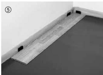
⑤ Starting in the right-hand corner of the room, align the boards of the first row with the tongue side parallel to the wall, and fix them in place with wall spacers as you proceed (always keep an expansion gap of 10--15 mm (3/8", -1/2") around perimeter).
