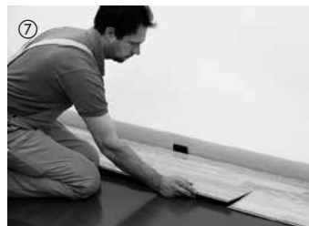
⑦ The next row is started with the leftover piece of the first row (short side offset of at least 50 cm). This considerably reduces waste. The rest of the installation is performed board-by-board. First, the boards are angled into the previous row along the long side by applying a small amount of force.
