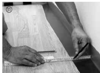
⑪ Cut to size and fit in the boards of the last row. Leave a gap of 10 to 15 mm between the boards and wall.
