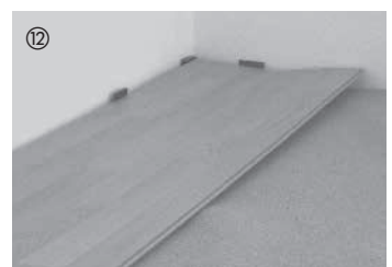
⑫ When you have interlocked the whole row on the long side and the short sides, you can lower it. Work from left to right.
