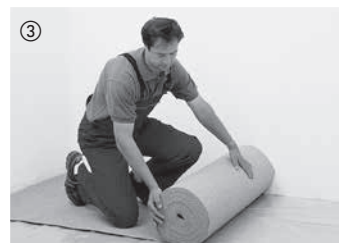
③ For sound insulation and to smooth out slight irregularities of the subfloor, unroll 2 mm thick cork underlay. Do not overlap. Our range of accessories also offers alternative insulation underlays. Asphalt-bitumen felt is not suitable for sound insulation. Do not use any additional insulation underlay when laying HARO laminate floor with Silent Pro ® .
