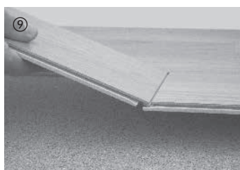
⑨ Insert the end of the next board of this row into the mating end of the board you just installed.
