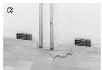
If radiator pipes protrude from the floor, drill or saw a cutout into the board (the size of the cutout depends on the radiator pipe and the required expansion space).
