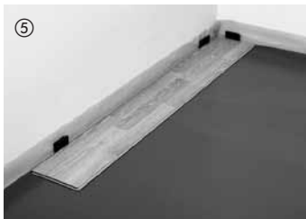
Starting in the right-hand corner of the room, align the boards of the first row with the tongue side parallel to the wall, and fix them in place with wall spacers as you proceed (always keep an expansion gap of 10–15 mm (3/8" - 1/2") around perimeter).
