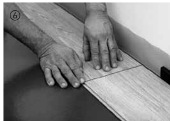
The remaining boards of the first row must be clicked in from above at the head ends into the previous boards. Pressure applied briefly to the side joint clicks in the board into the adjacent board. It is important to ensure that the first row is straight and exactly parallel to the wall. Cut the last board of the first row to size, leaving an expansion gap of 1015 mm (3/8" - 1/2") between the board and wall. Fit in the board and lay it flat.
