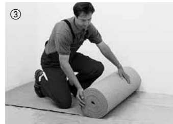
For sound insulation and to smooth out slight irregularities of the subfloor, unroll 2 mm thick cork underlay. Do not overlap. Our range of accessories also offers alternative insulation underlays. Asphalt-bitumen felt is not suitable for sound insulation. Do not use any additional insulation underlay when laying HARO laminate floor with Silent Pro®.
