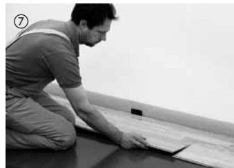
The next row is started with the leftover piece of the first row (short side offset of at least 50 cm). This considerably reduces waste. The rest of the installation is performed board-by-board. First, the boards are angled into the previous row along the long side by applying a small amount of force.
